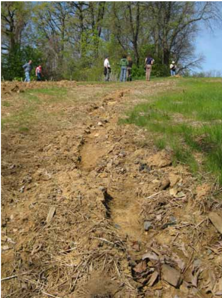
Erosion from the Rolling Meadow subdivision
